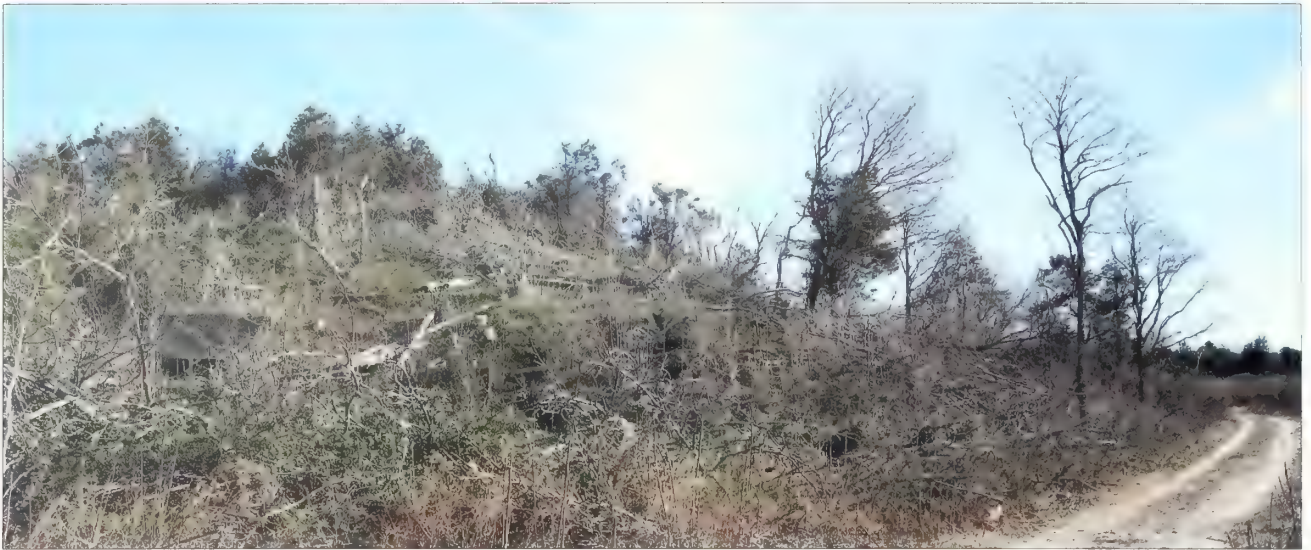
Figure 5.89. View looking east at southern end of Battery Mills. After recent cutting to manage invasive non-indigenous plant species, trunks, limbs, and other fallen debris were not removed. In order to safely and effectively permit future inspections and removals, the trunks and limbs have to be removed (Olmsted Center, January 2009).
